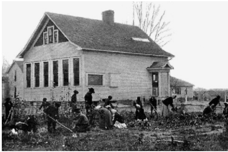
FIG. 15.—A rear view of the model rural school building at the Kirkville Normal.
