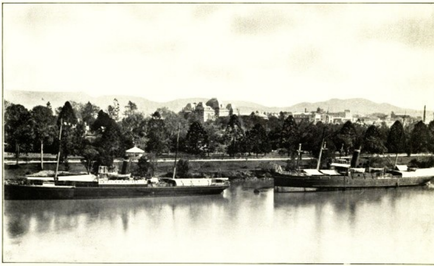
VIEW FROM RIVER TERRACE, BRISBANE
