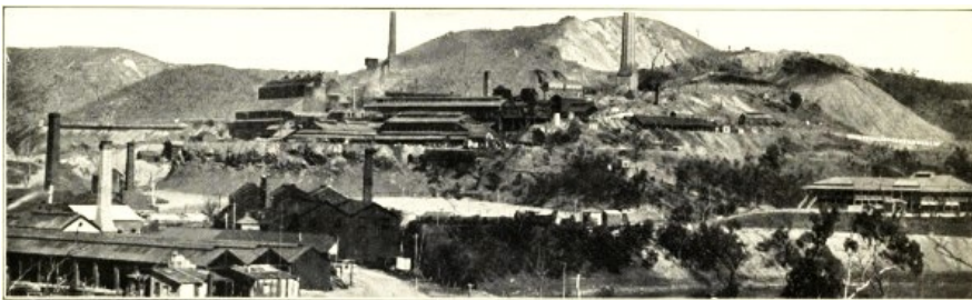
MOUNT MORGAN: GENERAL VIEW OF WORKS
