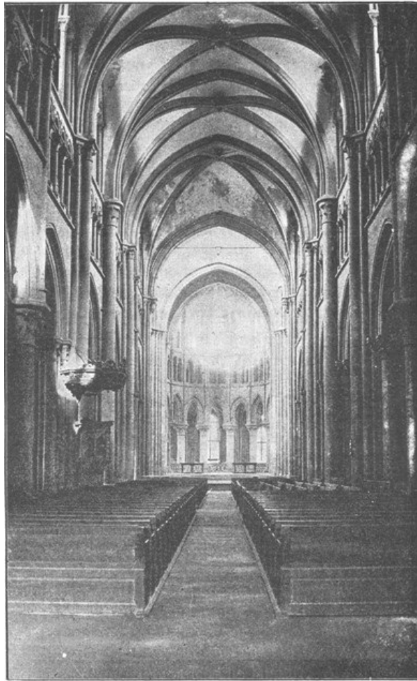
INTERIOR OF LAUSANNE CATHEDRAL. (From a Photograph.)
