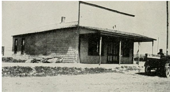
NOT A STORE BUT A CHURCH Christian Church at Des Moines, Union County.
