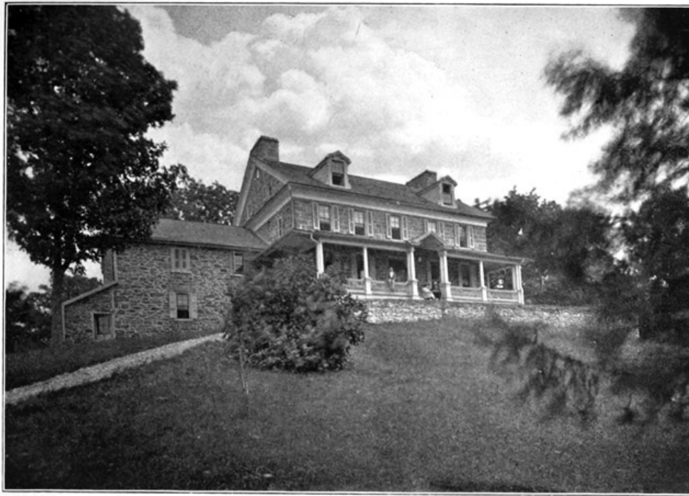
MILL GROVE MANSION ON THE PERKIOMEN CREEK. FROM A PHOTOGRAPH FROM W. H. WETHERILL, ESQ.
