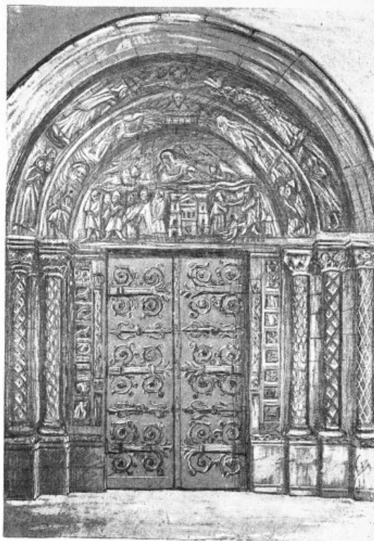
THE NORTH-WEST DOORWAY.
