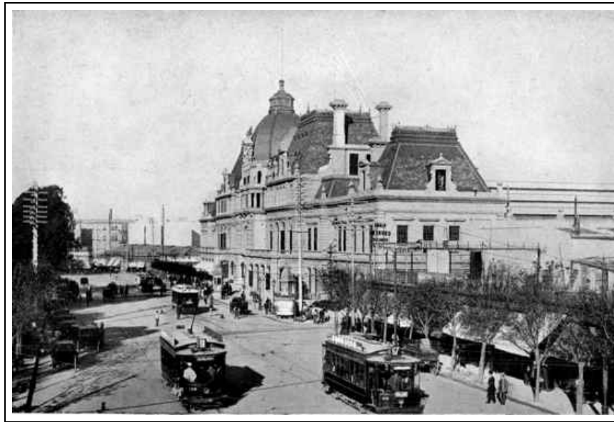
RAILWAY STATION, BUENOS AIRES GREAT SOUTHERN RAILWAY.
