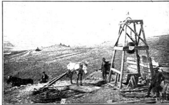
FIG. 84.—The horse lifts the bucket of ore.
