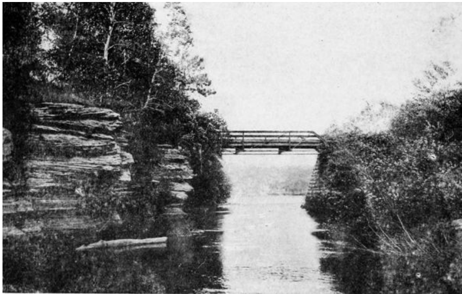
BRIDGE ACROSS DELL CREEK
