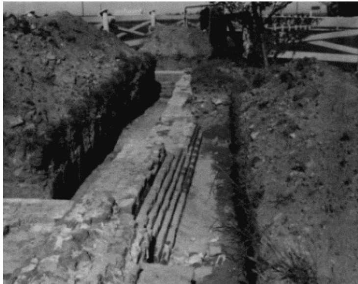
Figure 36.—SOUTH WALL OF STRUCTURE B, looking east. Base of veranda extends to bottom of picture at left. Molded-sandstone trim appears through brick rubble that has been attached to it, evidently as base for steps.
