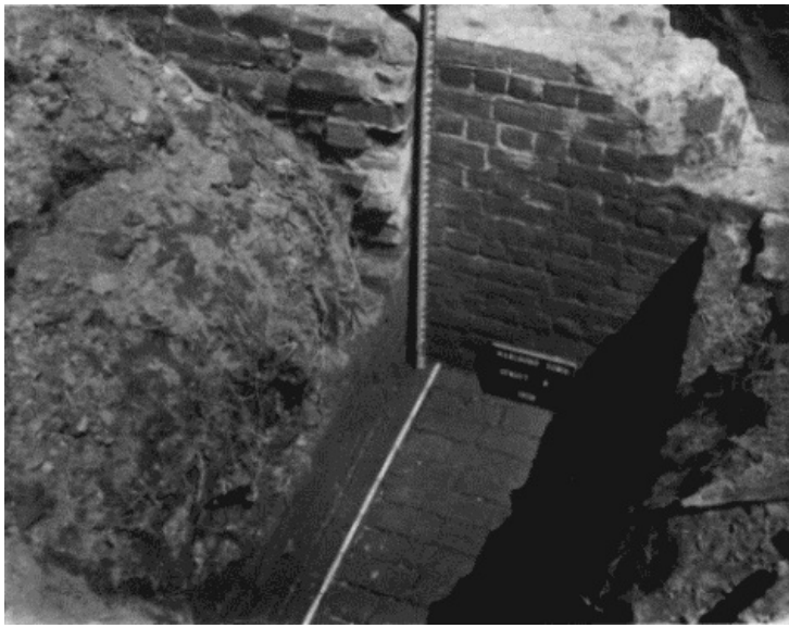
Figure 37.—CELLAR OF STRUCTURE B, showing remains of original cross wall at left and added cross wall at right. Mercer probably referred to the latter in 1749 in his account with Thomas Barry: “Underpinning and altering the cellar.”
