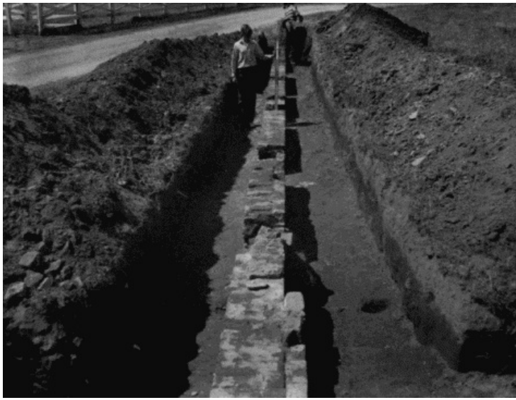
Figure 26.—WALL A-II. Breaks in wall date from subsequent placement of fence posts.
