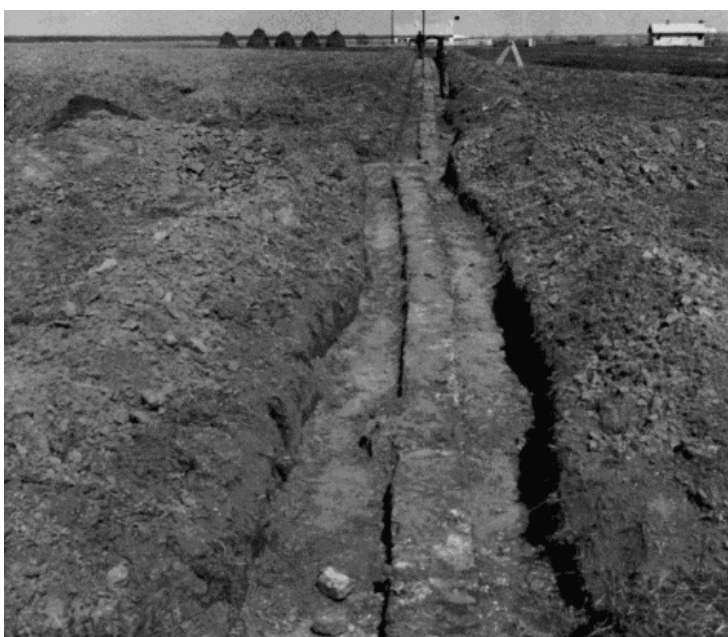
Figure 31.—WALL D, looking east toward Potomac River from Structure E (kitchen).
