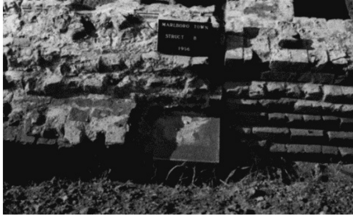
Figure 34.—SOUTHWEST CORNER OF STRUCTURE B. Piazza foundation extends to left, with red sandstone block at junction of piazza with main foundation. To the left of top of sign, molded red-sandstone trim can be seen which apparently surrounded the piazza. Bricks in front of trim appear to have been added later as step foundation. Brick buttressing of main-foundation footing appears at right.
