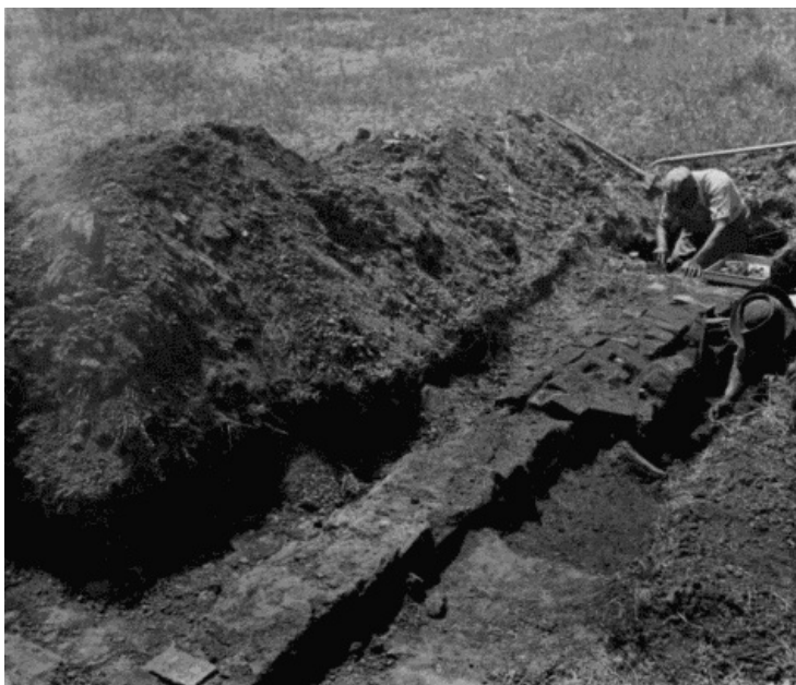
Figure 28.—WALL E, south of kitchen, showing gateway foundation.
