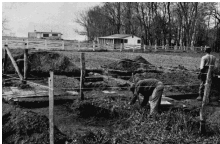
Figure 47.—FOUNDATION of Structure E (kitchen).
