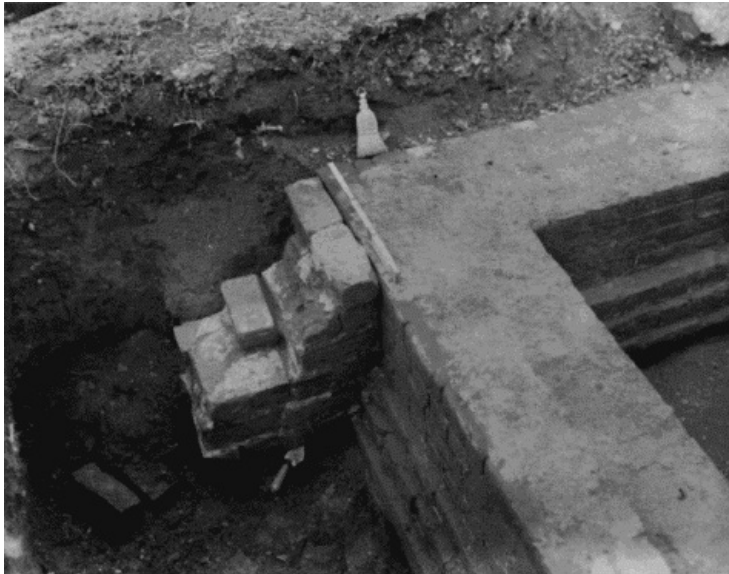
Figure 27.—JUNCTION OF WALL A-I with southeast corner of Structure B.
