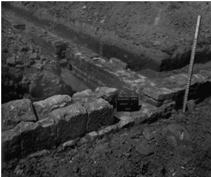
Figure 24.— JUNCTION OF STONE WALL A, running from creek side to this point, with brick Wall A-I at top left, Wall A-II at right.
