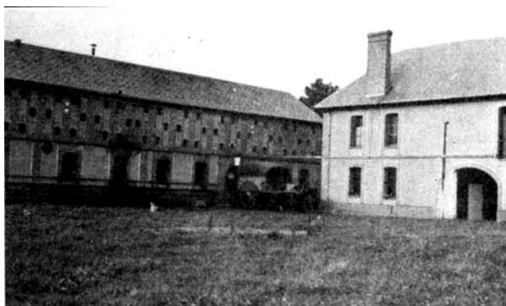
FIG. 22.—Camembert cheese factory at Lisieux, France. The square windows are seen in the second-floor rooms.
