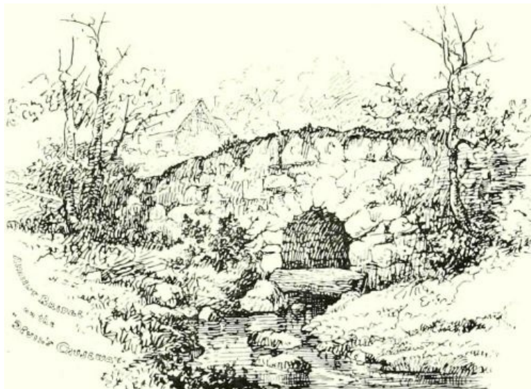
Ancient Bridge on the "Devil's Causeway."
