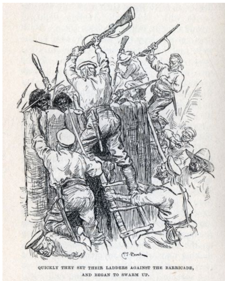
QUICKLY THEY SET THEIR LADDERS AGAINST THE BARRICADE, AND BEGAN TO SWARM UP.
