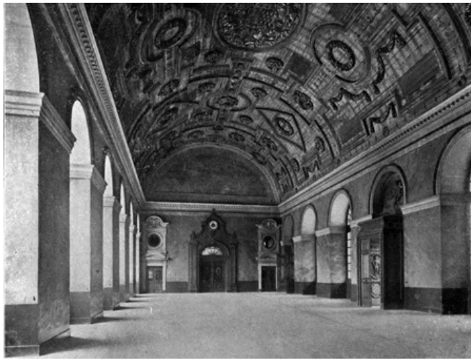
CEILING IN THE PALAIS DE JUSTICE, RENNES. LOUIS XIV PERIOD. (WOODEN CEILING IMITATING MASONRY VAULTING AND STUCCO ORNAMENTATION.)
