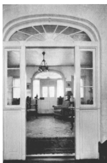
Figure 13. Detail, exterior door, north facade. 1969.
