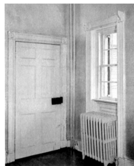
Figure 15. Detail, window and door, central first floor room. 1969.
