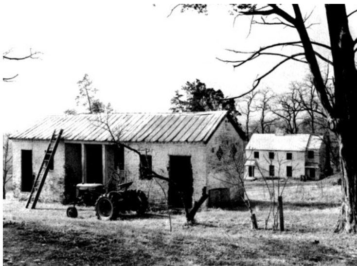
Figure 16. Necessary and tenant house from the icehouse, 1969. Photo by Wm. Edmund Barrett.
