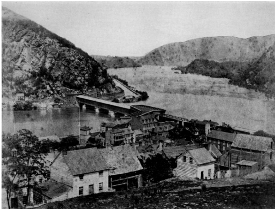
Figure 8.—THE BALTIMORE AND OHIO RAILROAD’S Potomac River crossing at Harpers Ferry, about 1860. Bollman’s iron “Winchester span” of 1851 is seen at the right end of Latrobe’s timber structure of 1836, which forms the body of the bridge. (Photo courtesy of Harpers Ferry National Historical Park.)
