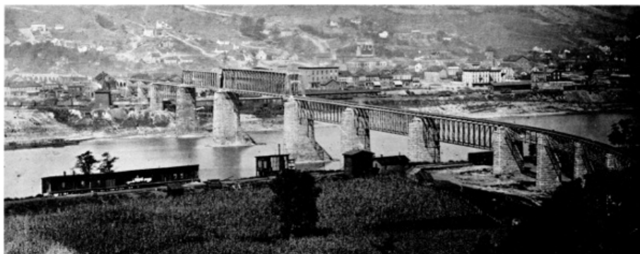
Figure 18. —OHIO RIVER CROSSING of the Baltimore and Ohio at Benwood, West Virginia, completed in 1870. Bollman deck trusses were used in the approaches on both sides. (Photo 693, Baltimore and Ohio Collection, Museum of History and Technology.)
