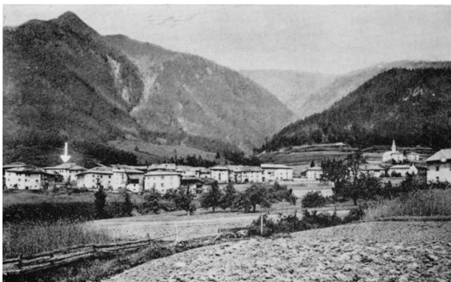
Figure 5.— THE VILLAGE OF MOCENIGO DI RUMO in the valley of the Non. Arrow points to Bertolla's home and workshop at far left.
