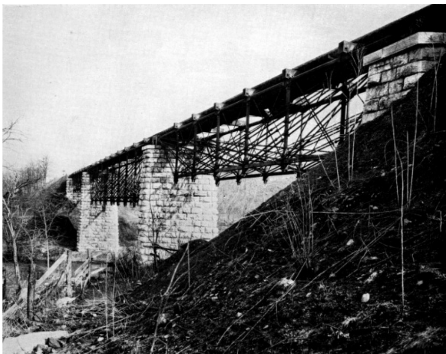
Figure 22.—BOLLMAN DECK TRUSSES in the North River Bridge built in 1873 at Mount Crawford, Virginia, on the Valley Railroad of Virginia (B. & O.). Each end span is 98 ft. 6 in.; the river span is 148 ft. 9 in. (Photo 756, Baltimore and Ohio Collection, Museum of History and Technology.)
