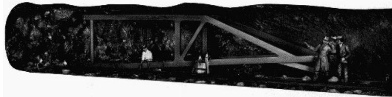
Figure 3.—HOOSAC TUNNEL. WORKING OF LATER STAGES with Burleigh pneumatic drills mounted on carriages. The bottom heading is being drilled in preparation for blasting out with nitroglycerine. MHT model — ½" scale. (Smithsonian photo 49260-M.)
