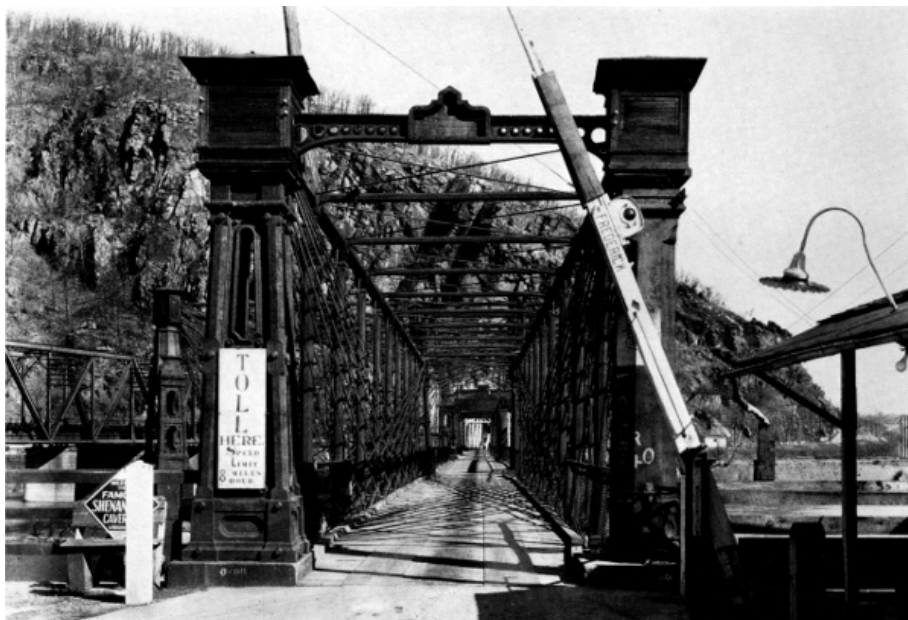
Figure 21.—THE HARPERS FERRY BRIDGE toward the end of its career, carrying a common road over the Potomac. The westernmost line of trussing and span no. 1 had been removed long before. View through the Winchester span looking toward Maryland in 1933. (Photo courtesy of Harpers Ferry National Historical Park.)
