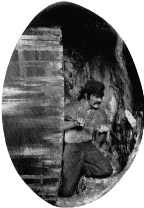
Figure 31.—EXCAVATION IN FRONT OF SHIELD, Tower Subway. This was possible because of the stiffness of the clay encountered. MHT model—front of model shown in fig. 29. (Smithsonian photo 49260-A.)
