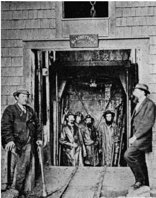
Figure 7.—HOOSAC TUNNEL. GROUP OF MINERS descending the west shaft with a Burleigh drill. (Photo courtesy of State Library, Commonwealth of Massachusetts.)
