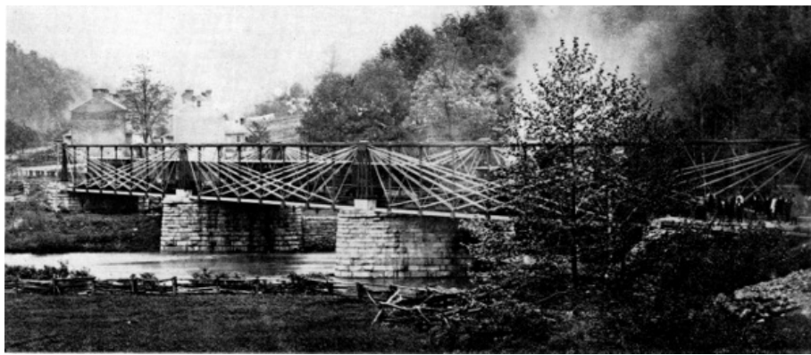
Figure 9.—BOLLMAN SKEW BRIDGE at Elysville (now Daniels), Maryland, built in 1853-1854. (Photo courtesy of Maryland Historical Society.)
