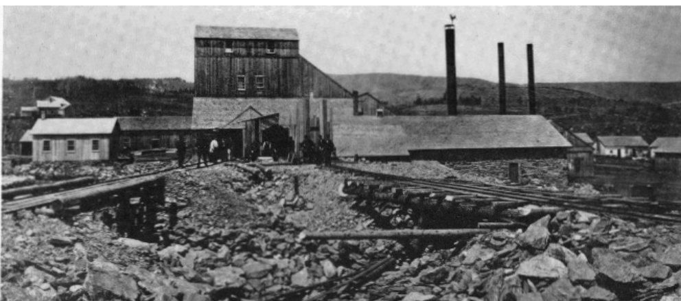
Figure 12.—WORKS AT THE CENTRAL SHAFT, HOOSAC TUNNEL, for hoisting, pumping and air compressing machinery, and general repair, 1871. (Photo courtesy of State Library, Commonwealth of Massachusetts.)
