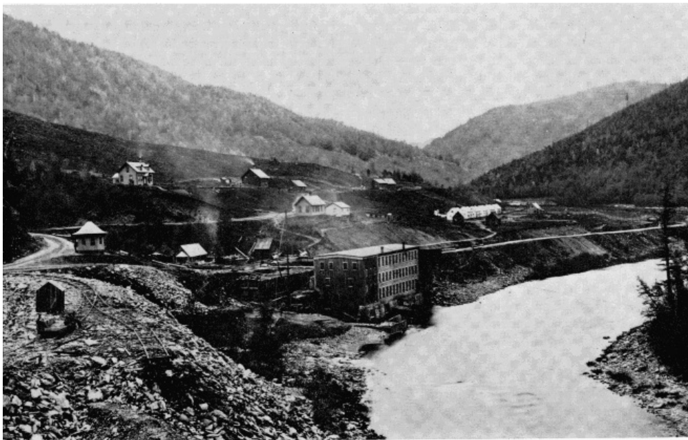
Figure 13.—HOOSAC TUNNEL. AIR-COMPRESSOR BUILDING on Hoosac River near North Adams. The compressors were driven partially by waterpower, derived from the river. (Photo courtesy of State Library, Commonwealth of Massachusetts.)
