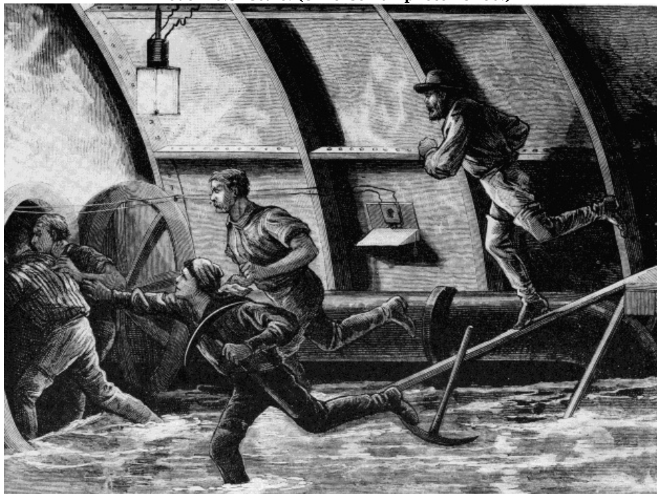
Figure 40.—ARTIST'S CONCEPTION OF MINERS escaping into the air lock during the blowout in Haskin's tunnel.
