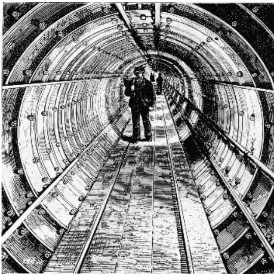
Figure 32.—INTERIOR OF COMPLETED TOWER SUBWAY. (THORNBURY, Old and New London , 1887, vol. 1, p. 126.)
