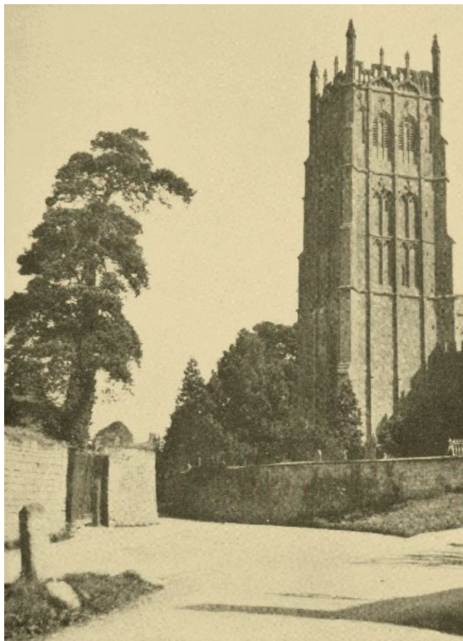
TOWER OF CHIPPING CAMPDEN CHURCH
