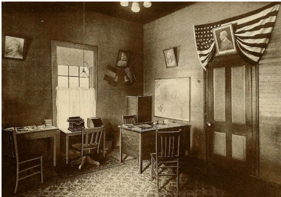
INTERIOR WAR SERVICE STATION, Riverview
