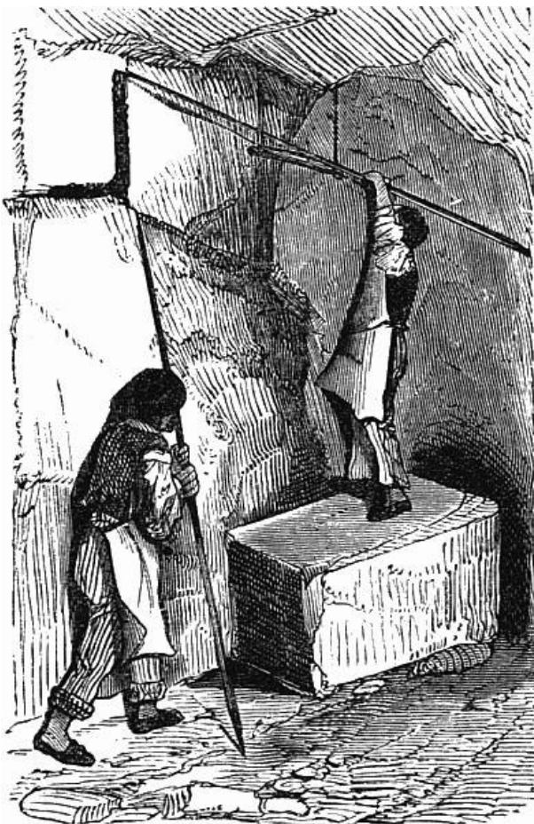
Fig. 24. Extracting the stone in subterranean quarries.
