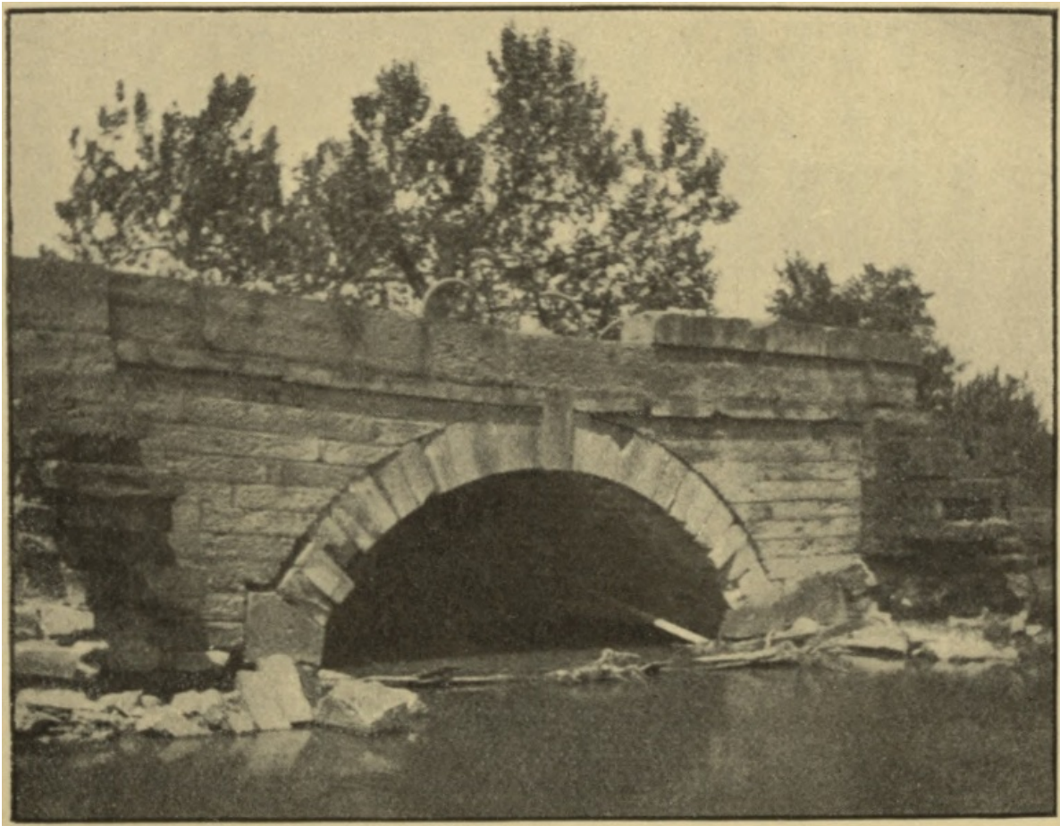
CULVERT ON THE CUMBERLAND ROAD IN OHIO
