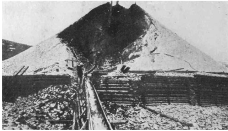
SLUICING THE WINTER DUMP AT FAIRBANKS
