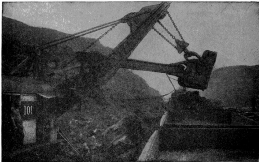
STEAM SHOVEL LOADING ROCK
