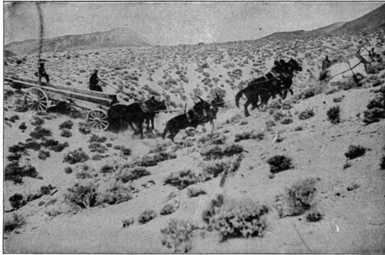
THIS PICTURE SHOWS THE DIFFICULTIES ENCOUNTERED IN HAULING POLES IN A MOUNTAINOUS SECTION ALONG THE TRANSCONTINENTAL LINE OF THE BELL SYSTEM
