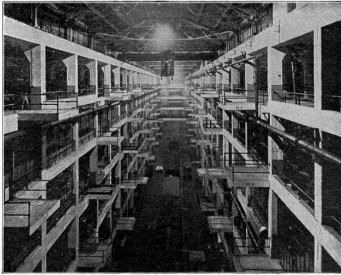
CRANEWAY, SHOWING LOADING PLATFORMS
