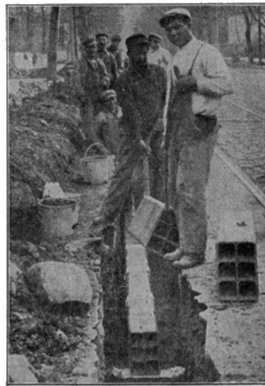
TILE CONDUITS USED IN AMERICAN UNDERGROUND CONSTRUCTION
