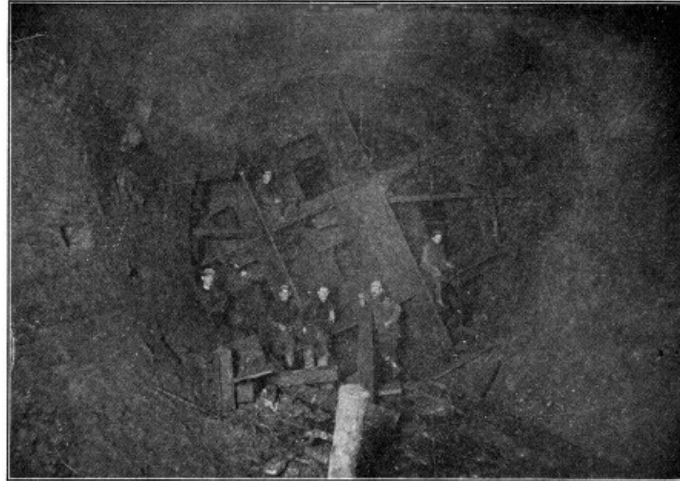
CUTTING EDGE OF SHIELD IN NORTH TUNNEL
