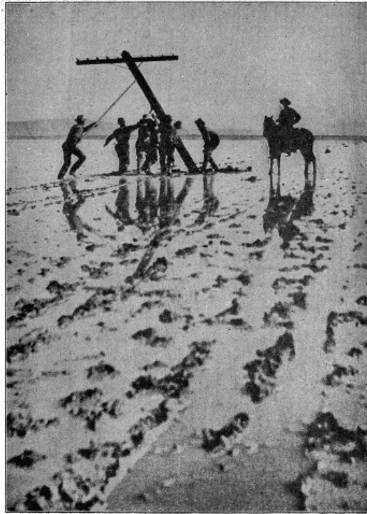
SETTING POLES ACROSS A SHALLOW LAKE IN NEVADA DURING THE CONSTRUCTION OF THE TRANSCONTINENTAL LINE OF THE BELL SYSTEM
