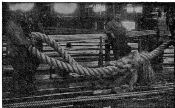
SIXTEEN-INCH TOWLINE WITH EYE SPLICE
