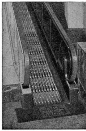
A CLEAT TYPE ESCALATOR, SHOWING THE HARDWOOD CLEATS USED IN PLACE OF STEPS
