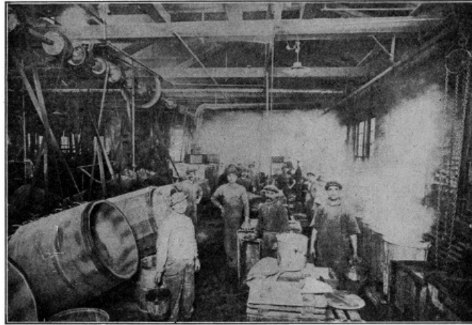
THE WHITENING ROOM, WHERE THE PINS ARE CLEANED AND PLATED
