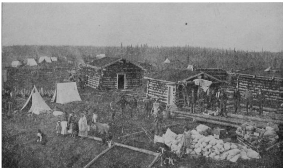
SUPPLY STATION FOR CIRCLE CITY.
