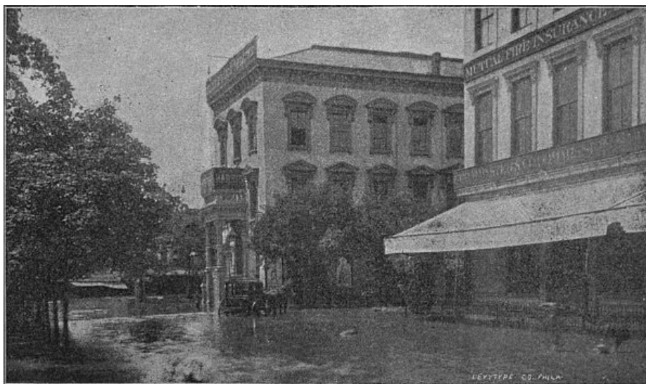
SEVENTH STREET, WASHINGTON, DURING THE FLOOD.
