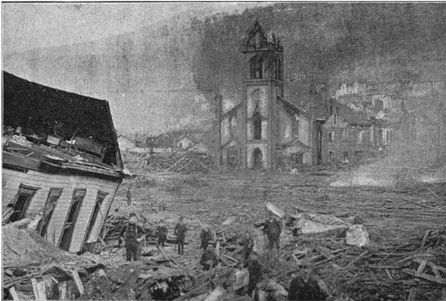
RUINS FROM SITE OF THE HURLBURT HOUSE.
