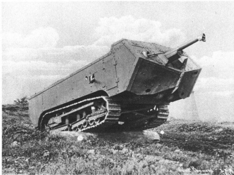
A new type of tank made for the French Army (© Underwood)
