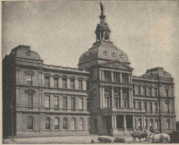
THE GOVERNMENT BUILDING, PRETORIA, TRANSVAAL
