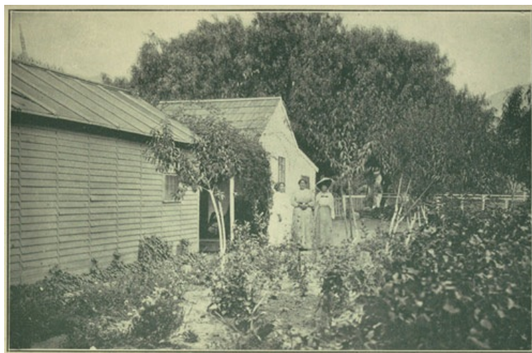
One of the Portable Houses bought by the U. S. Indian Department. The rear house was erected by the Indians
