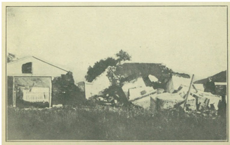
The Ruins of the Pala Campanile, After Its Fall in January, 1916.
