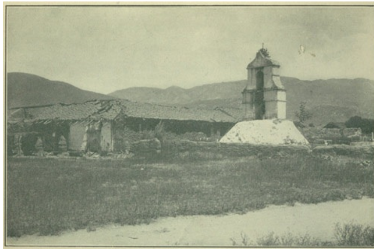
The Pala Chapel and Campanile Before the Restoration.
