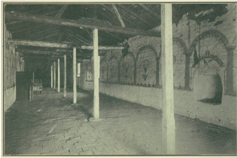
Interior of Pala Chapel Before the Restoration, Showing the Old Indian Mural Decorations.
