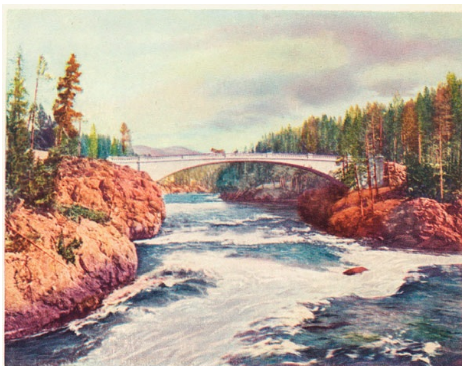
Bridge above The Rapids
