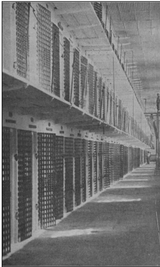
CORRIDOR IN CELL HOUSE.
