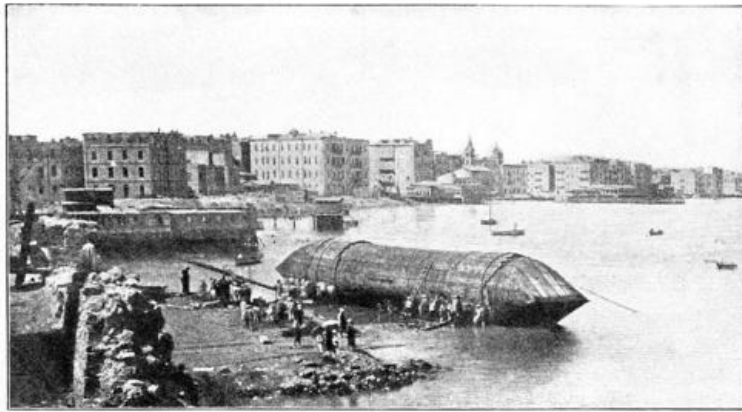
From a] [Photo. REPAIRING THE HOLE MADE BY THE ROCK.
