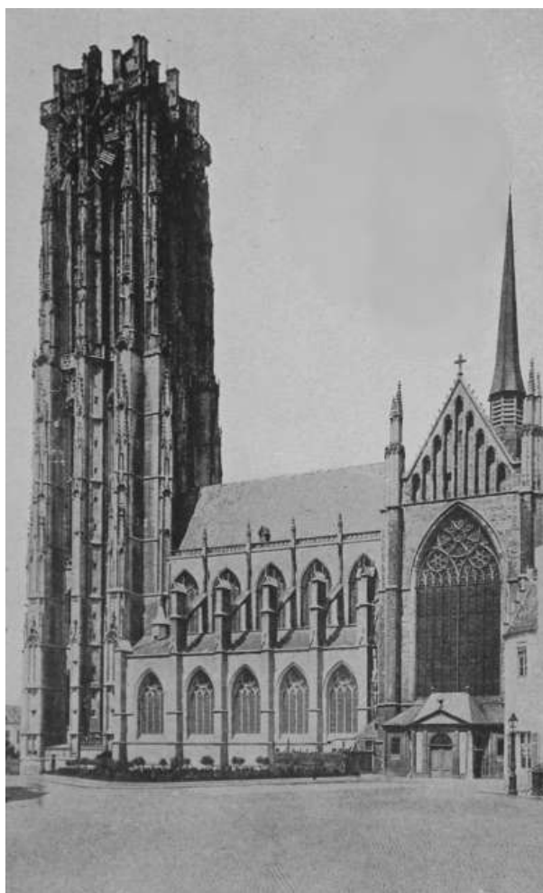
CATHEDRAL OF ST. ROMBAUT. MALINES.
