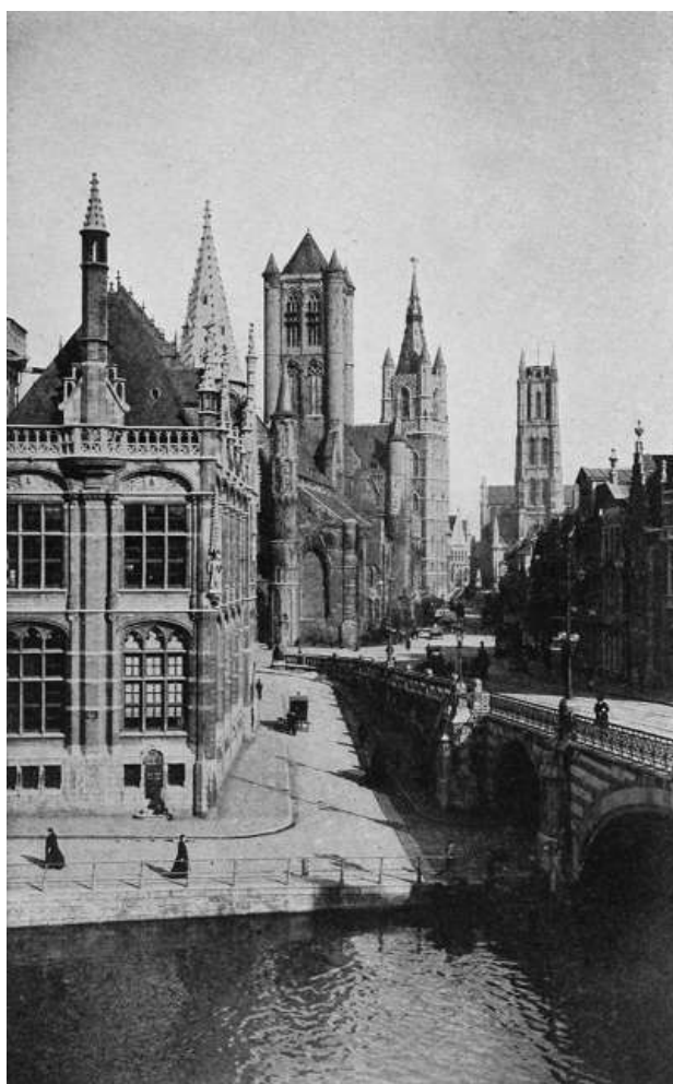
POST OFFICE, CHURCH OF ST. NICHOLAS, BELFRY AND CATHEDRAL, GHEENT.
