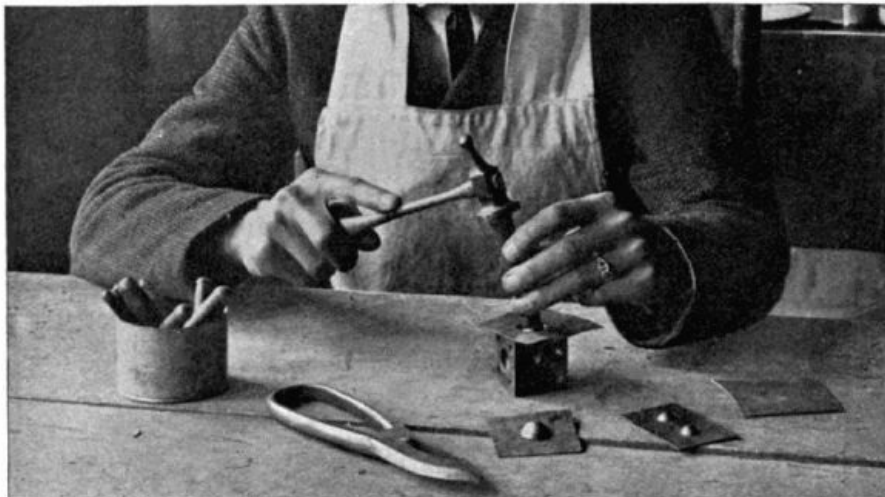
FIGURE 29. Dapping tools in use.
