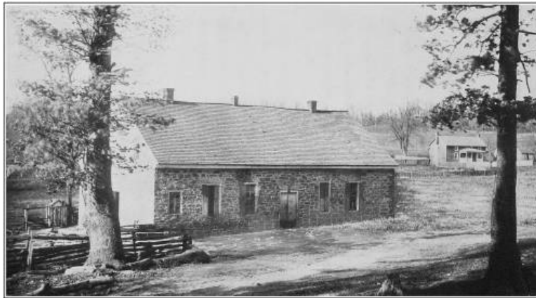
NEW PROVIDENCE CHURCH, ROCKBRIDGE COUNTY, VIRGINIA
