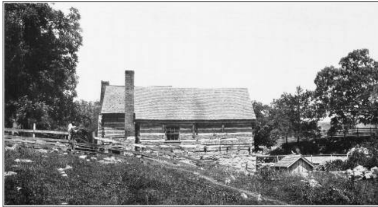
OLD BLACKSMITH SHOP ON WALNUT GROVE FARM, VIRGINIA
