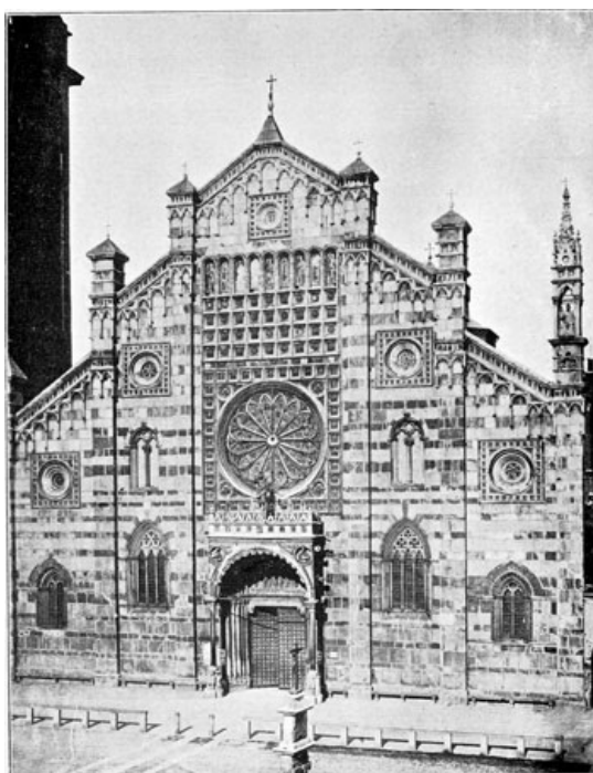
FAÇADE OF MONZA CATHEDRAL. RESTORED 14TH CENTURY.
