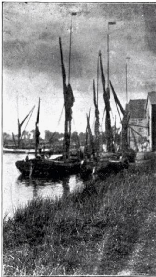
BARGES AT AN ESSEX MILL
