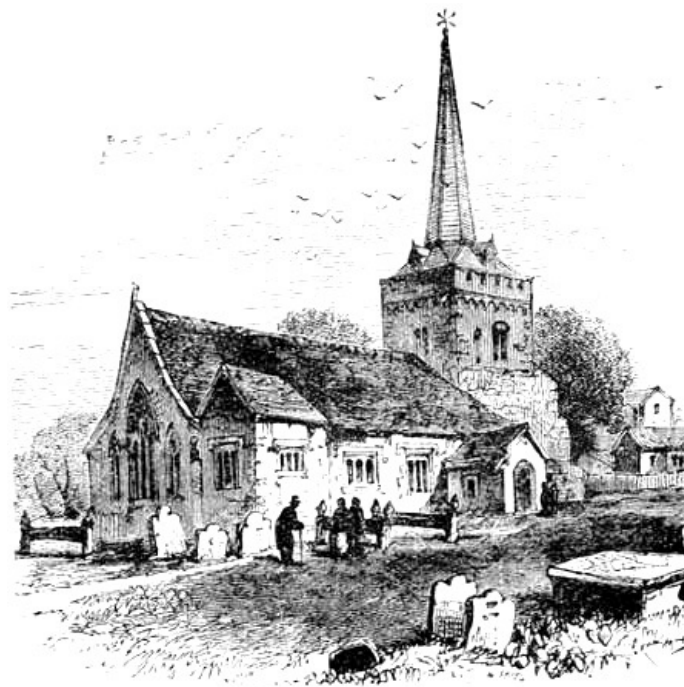
Cuckfield Church, Sussex—before restoration.
