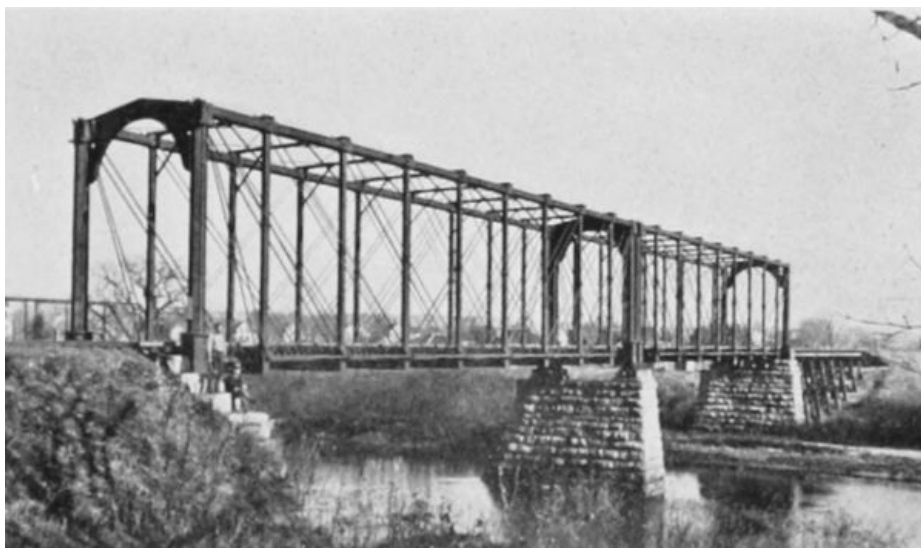
BRIDGE OVER WAPSIE AT CENTRAL CITY
