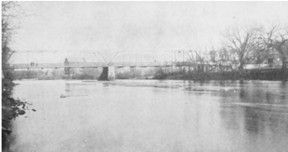
UPPER WAGON BRIDGE, CENTRAL CITY
