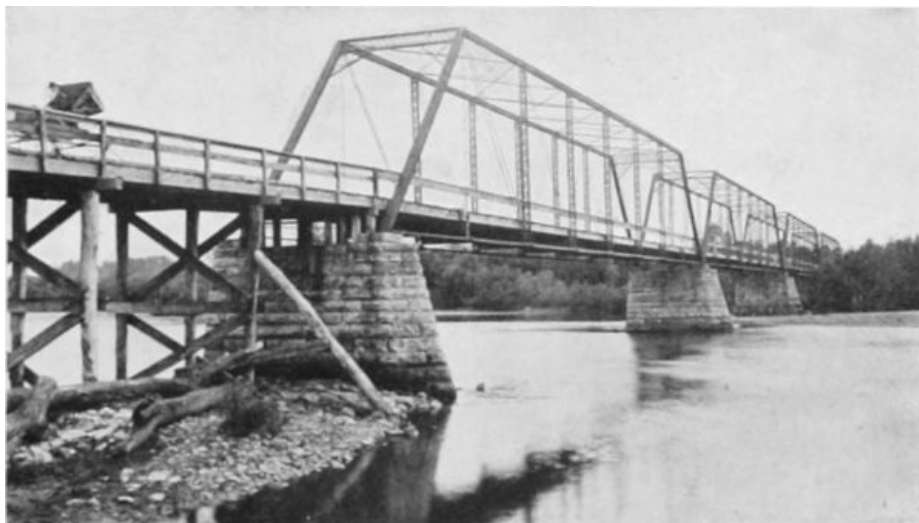
BRIDGE OVER CEDAR RIVER AT CENTER POINT
