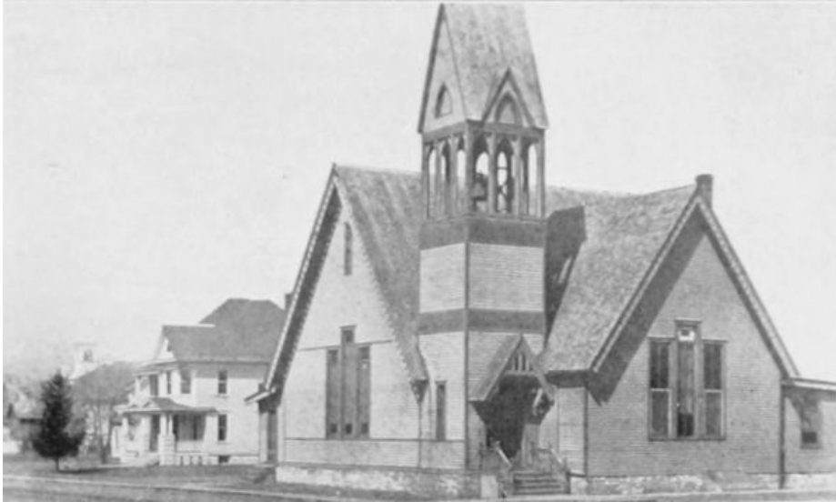
CONGREGATIONAL CHURCH, CENTRAL CITY
