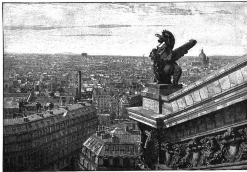
Mont Valérien and the Arc de Triomphe.—Church of St. Augustine. VIEW FROM THE ROOF OF THE OPERA HOUSE.
