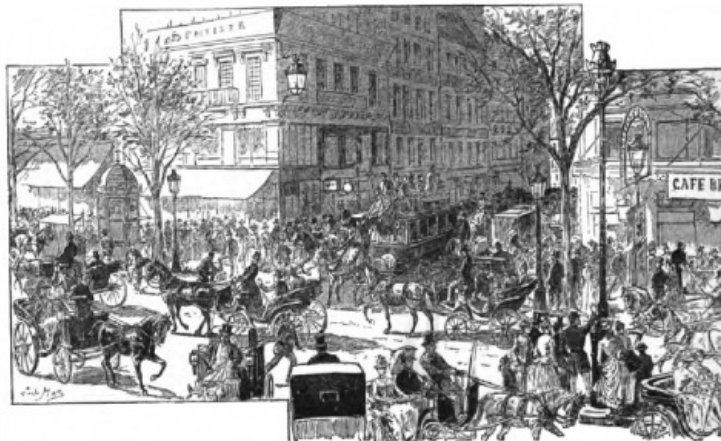
JUNCTION OF GRAND BOULEVARDS AND RUE AND FAUBOURG MONTMARTRE.
