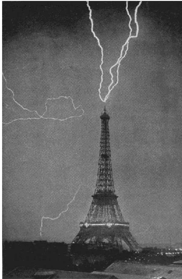
THE EIFFEL TOWER AS A COLOSSAL LIGHTNING CONDUCTOR. Photograph taken June 3, 1902, at 9.20 p.m., by M. G. Loppé. Published in the Bulletin de la Société Astronomique de France (May, 1905)
