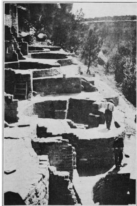
TERRACES AT SOUTHERN END, AFTER REPAIRING
