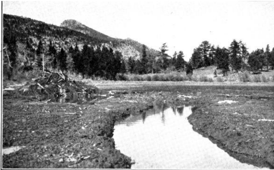
SECTION OF A 750-FOOT CANAL AT LILY LAKE Here five feet wide and three feet deep
