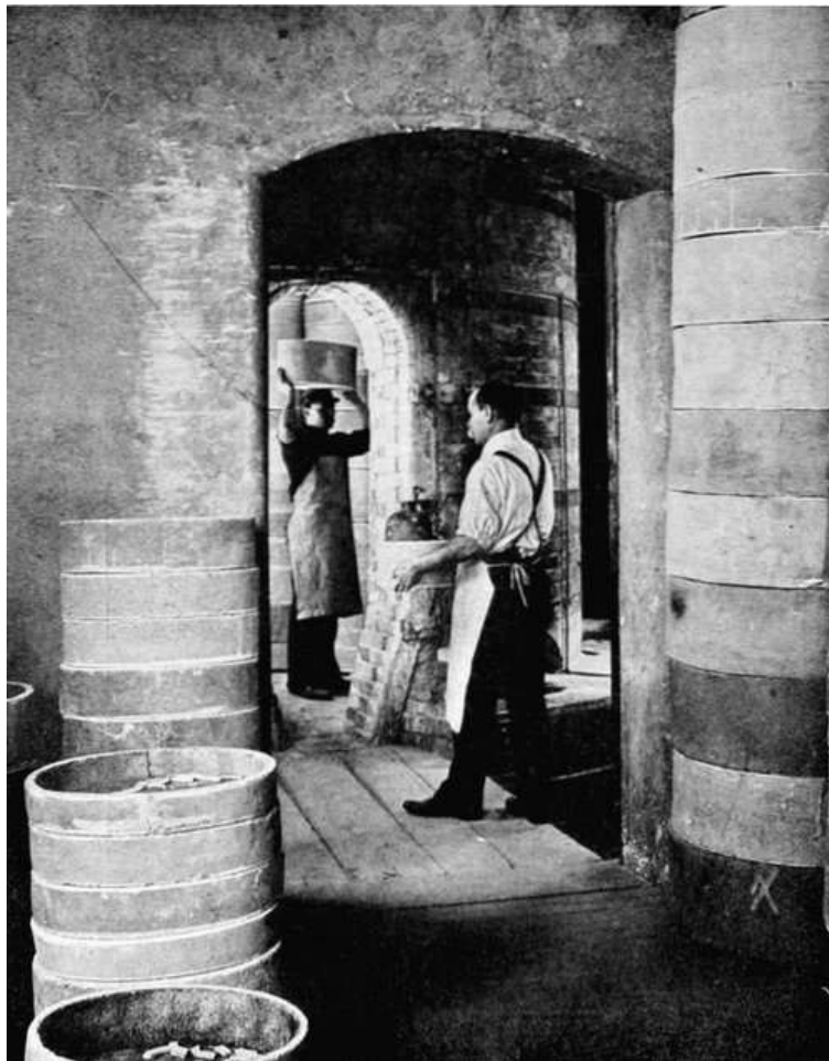
FIGURE 282.—Stacking the Kiln
