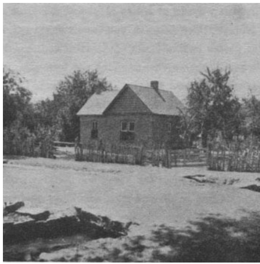
MORMON HOUSE AND IRRIGATION DITCH
