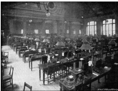
A PORTION OF A TELEGRAPHIC OPERATING ROOM AT THE GENERAL POST OFFICE, LONDON.
