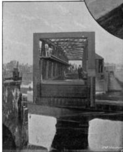
From a Photograph [by E. Ward, Manchester. BARTON AQUEDUCT.
