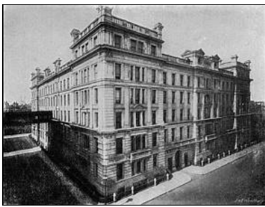
GENERAL POST OFFICE—NEW NORTH BUILDING.
