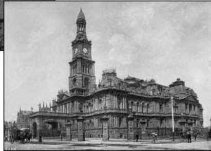
THE TOWN HALL, CENTENNIAL HALL, AND CATHEDRAL, SYDNEY.
