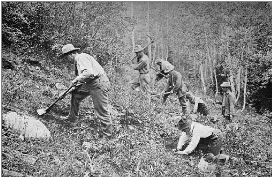
Figure 28. A planting crew at work setting out small trees. The man ahead digs the hole, and the man behind plants the tree. Wasatch National Forest, Utah
