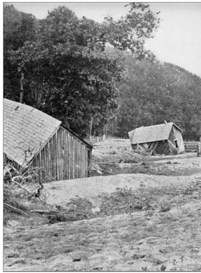
Figure 49. Wrecked farm buildings due to flood of May 21, 1901, Nolichucky River, near Erwin, Tenn. This is one result of denuding the Appalachian Mountains of their forest cover.
