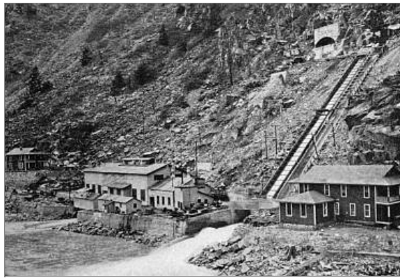
Figure 78. The power plant of the Colorado Power Company, on the Grand River, Holy Cross National Forest, Colorado. Every fiscal year there is a substantial increase in water power development on the National Forests.
