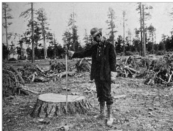
Figure 69. View showing the Forest Service method of piling the brush and debris after logging, and also how stump heights are kept down to prevent waste. New Mexico.
