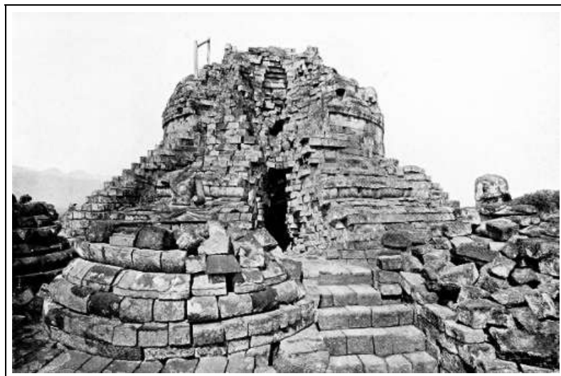
XXXIX. THE DAGOB OF THE BORO BUDOOR BEFORE ITS RESTORATION (C. Nieuwenhuis.)
