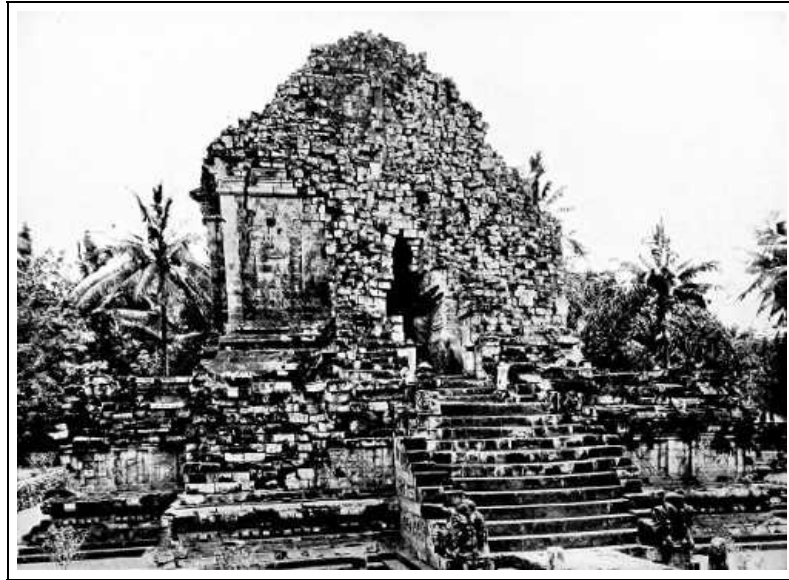
XXIII. CHANDI MENDOOT BEFORE ITS RESTORATION (Cephas Sr.)
