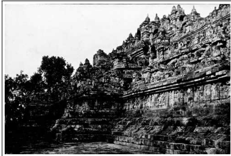
XXVIII. BASE OF THE BORO BUDOOR SHOWING THE (FILLED UP) LOWEST GALLERY (C. Nieuwenhuis.)
