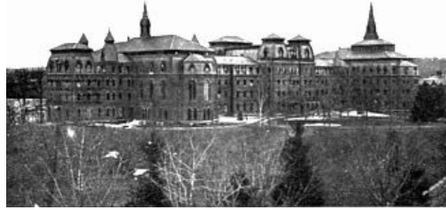
College Hall, destroyed by fire in 1914
