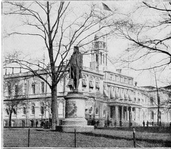
... City Hall with its grateful lack of height ...
