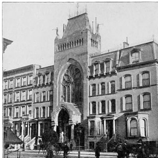
The Church of the Heavenly Rest.
