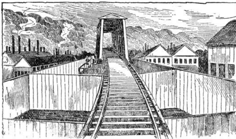
PEMICKEY TRACK IN THE MILL YARD.
