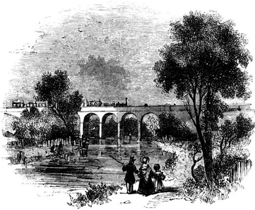
VIADUCT, NEAR WATFORD, BIRMINGHAM RAIL-ROAD.
